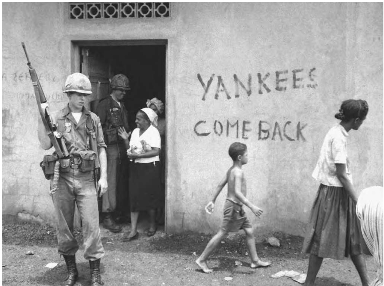
A U.S. Army soldier patrols the streets of Santo Domingo, Dominican Republic, on 9 May 1965 during a period of civil unrest. The message "Yankees come back" is scrawled on the wall of a building where food is being distributed. (National Archives and Records Administration)
