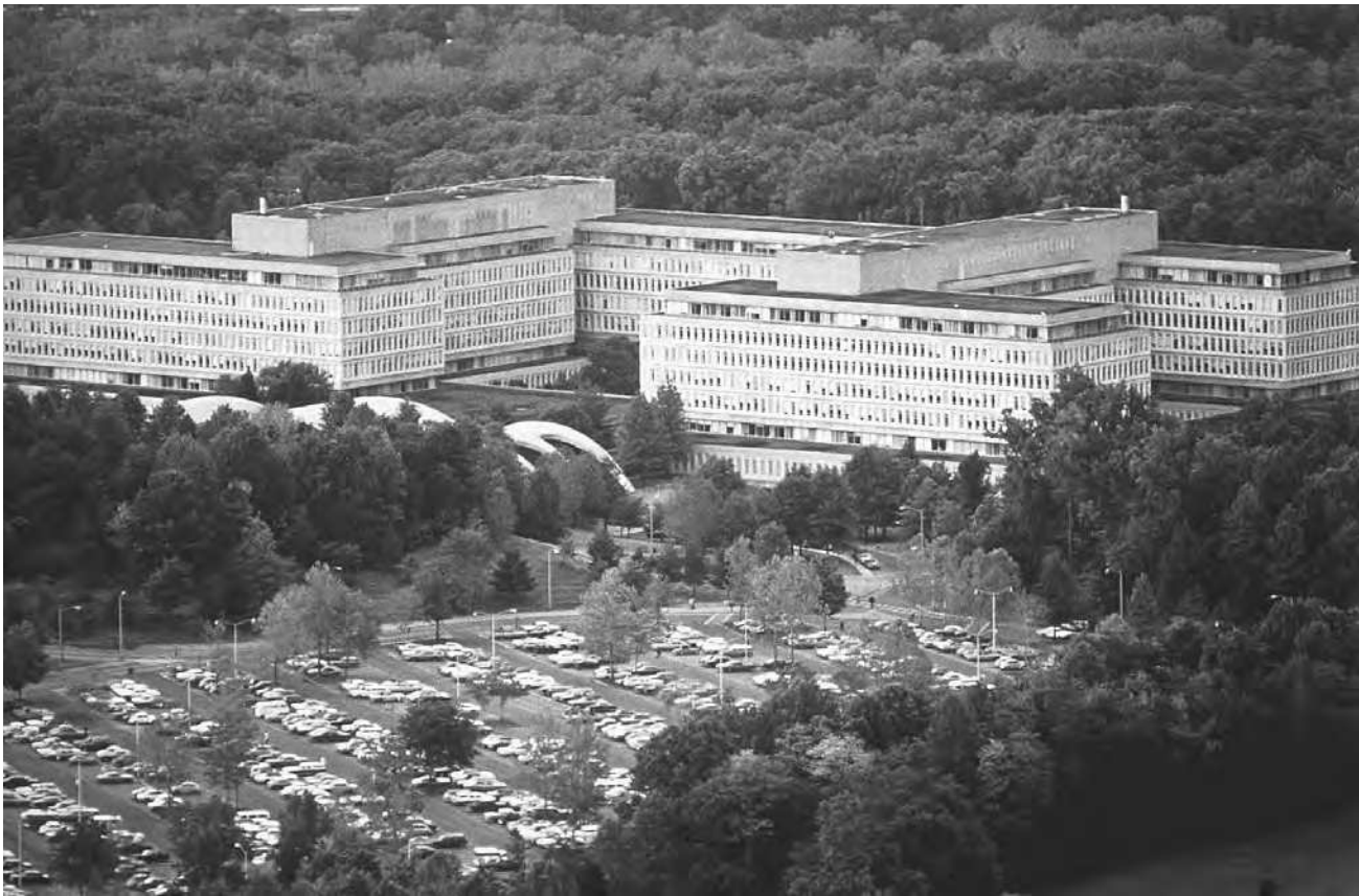
Central Intelligence Agency headquarters, Langley, Virginia. (National Archives and Records Administration)
