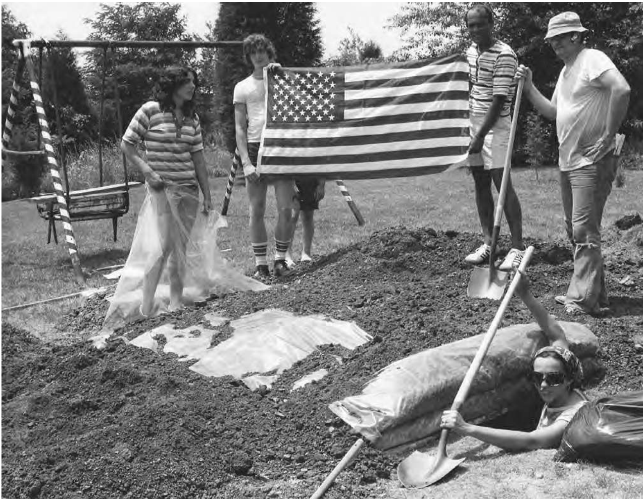
Fallout shelter being dug by a family near Mechanicsburg, Pennsylvania. The program was funded by the Defense Civil Preparedness Agency. Under this program, families were paid to build various kinds of expedient fallout shelters (fast shelters that could be built in a nuclear emergency) to find out how quickly the shelters could be built and to test the adequacy and clarity of shelter plans. (National Archives and Records Administration)
