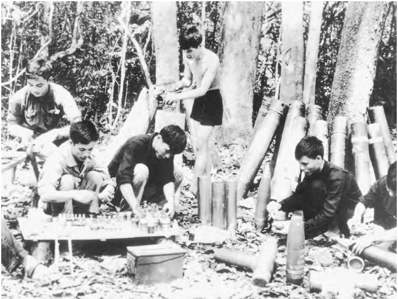
During the Vietnam War, the Viet Cong constructed antipersonnel mines from such materials as artillery and mortar shells, cartridge cases, and pipe. U.S. forces sustained significant casualties from these weapons. (U.S. Army Center of Military History)
